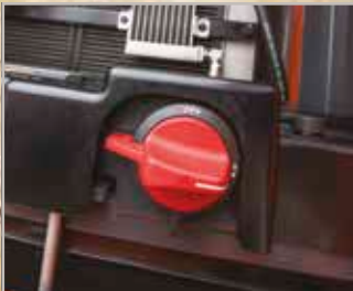
Battery cut-off switch
